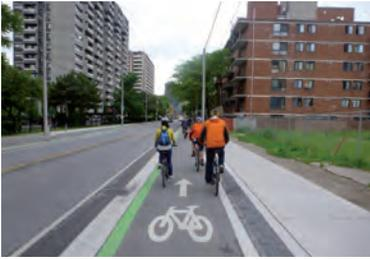
Operating space is required beyond the edge of the bikeway especially for cyclists when passing
